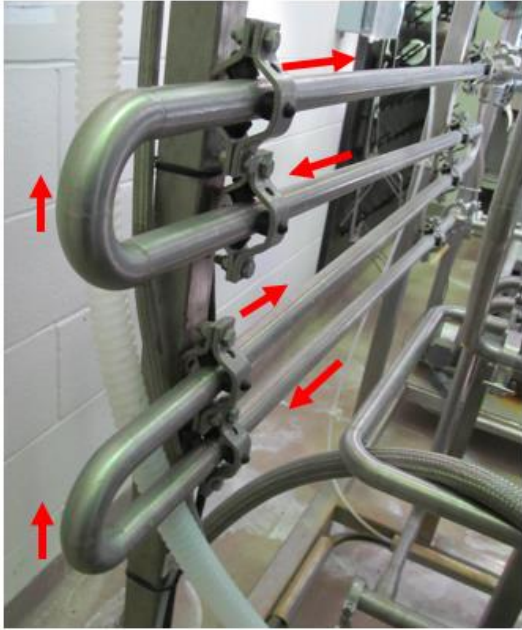
Figure 6-30: Holding tube section of heat exchanger system. Arrows indicate direction of fluid flow.
