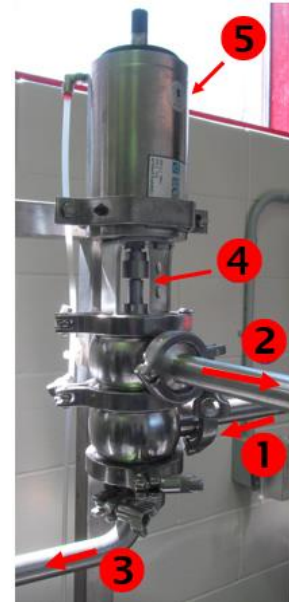
Figure 6-31: Flow diversion valve (numbered items are explained in text).
